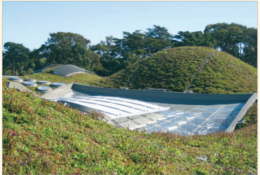
This green roof on the California Academy of Sciences building in San Francisco includes native plants that are well adapted to long, dry summers.
