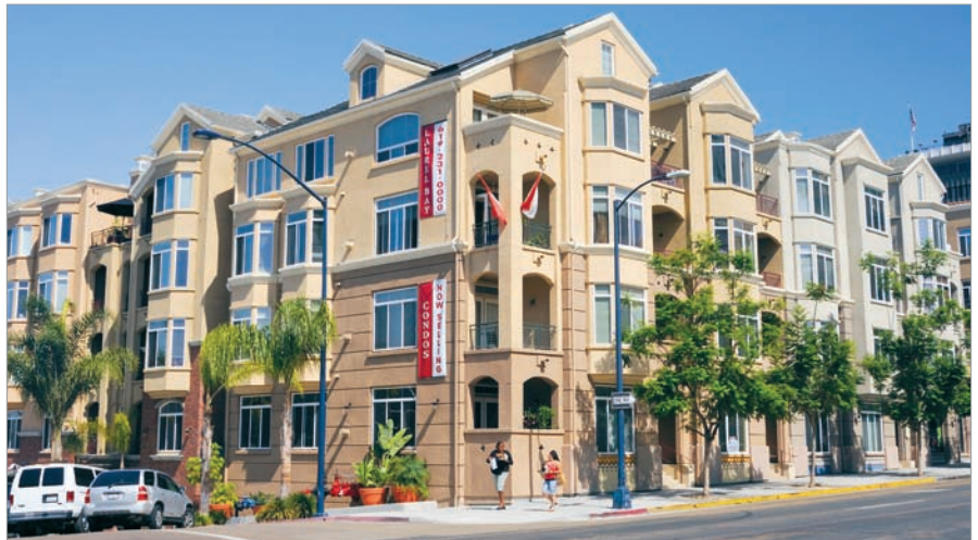
A residential development in San Diego uses varying wall planes and bay windows to create a rhythm on the building's façade.
