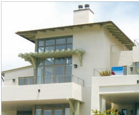
Visible rafter tails provide details that strengthen the roofline of this building in Coronado.
