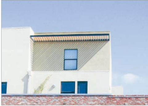
A projecting feature on this building in Emeryville, California, provides shade for a window.
