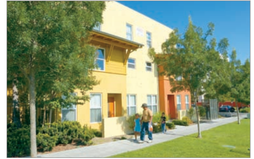
Landscape design enhances public space and softens the edges of these apartments in San Diego.
