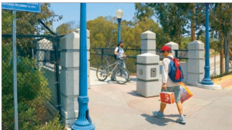
A pedestrian and bicycle overpass in San Diego creates a connection across a canyon.
