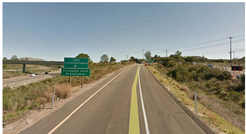
I-8 East Willows Road EB off-road signage
