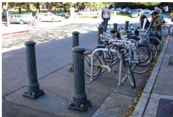
On-Street Bike Parking with Inverted U Racks
